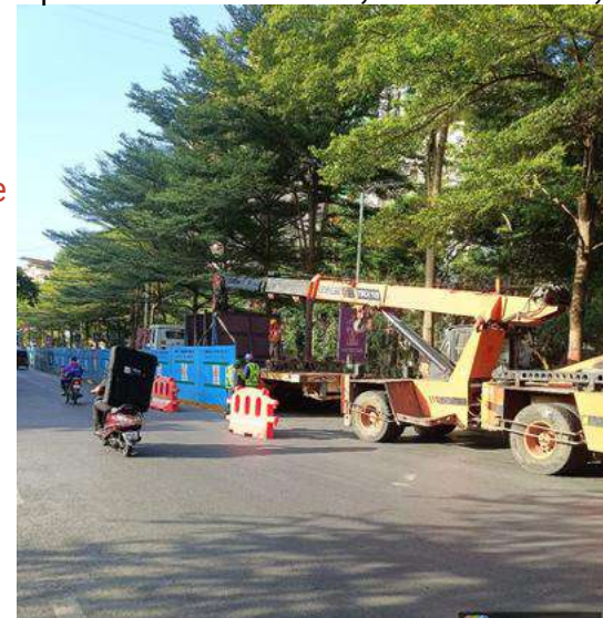
Gladys Alvares Marg, Ring Metro Work closing 1 lane completely bang at start of monsoon
